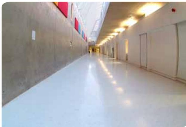
Isogran is a polymer modified granolithic wearing screed providing a tough, hard wearing floor, ideal for heavy duty use in buildings such as workshops, plant rooms, store rooms and service corridors.
